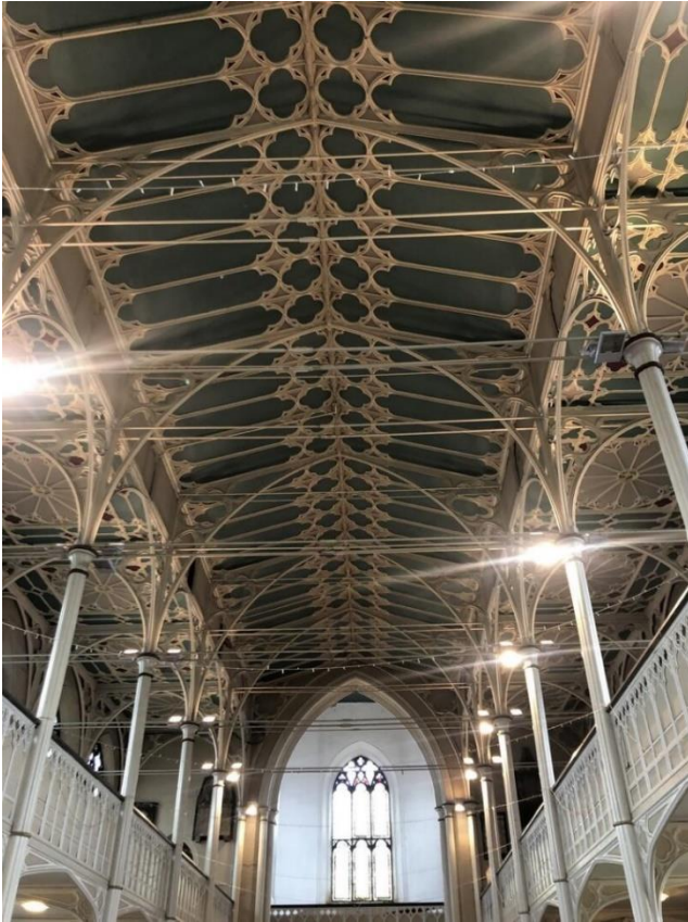
The interior of the cast iron church, showing the groundbreaking pre-fabricated structure.
